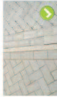
Use of porous paving in tertiary street layout along services corridor must be designed to match neighbouring paving (refer to traffic section page 4.6)
